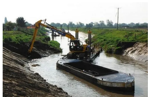
River dredging operations (source: www.indiamart.com)
