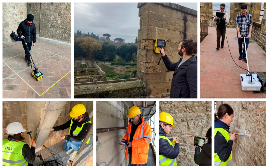
Figure 7. The diagnostic campaign conducted on the construction.
