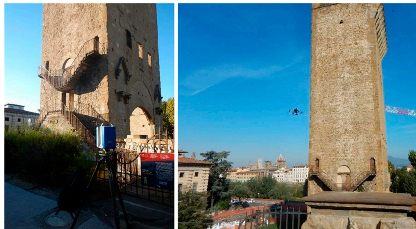
Figure 5. The digital survey was performed using 3D laser scanners and a drone.
