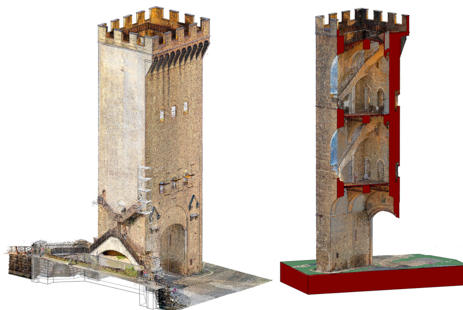
Figure 11. The point cloud overlapping the three-dimensional model of the Tower.
