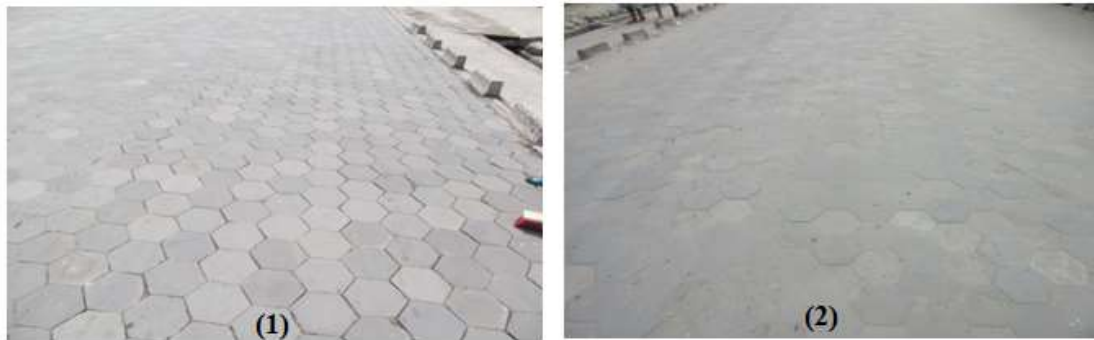
Fig. 4. View of the paving stones at the start of installation (1) and after 8 years (2)
