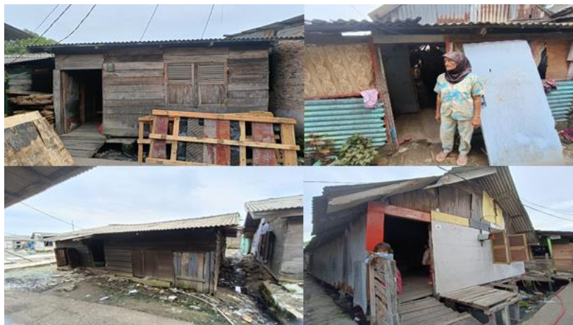
Fig. 2. House condition temporary
