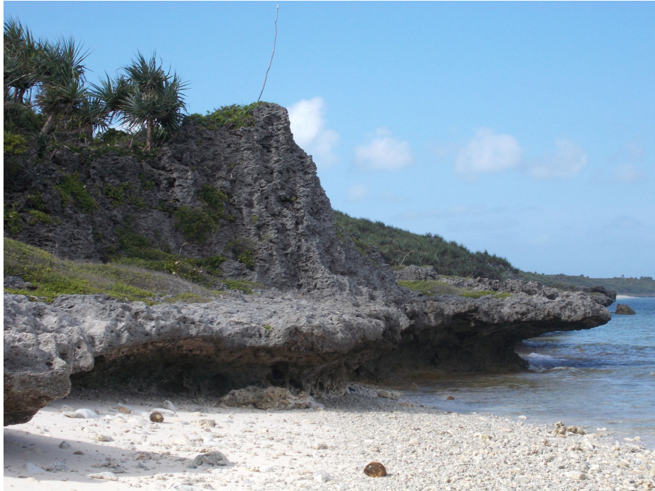
Figure 40. The present under-cut notch at HTL and a very distinct shore-cut platform above at about +70 - 80 cm (above HTL). It is quite moderately weathered and is most likely to correlate to the +70 cm terrace in Site 17 [9].
